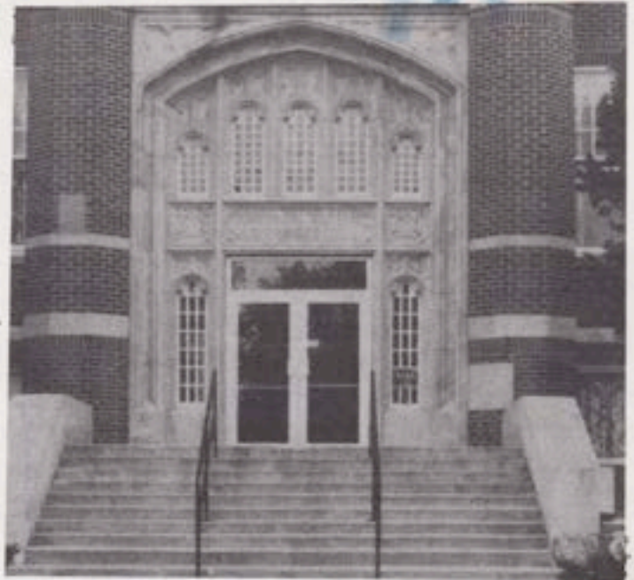
Entrance was blocked while the construction progressed.
